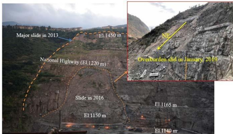
Fig. 1. Slide boundary of right abutment of PPHA-I, Dam
